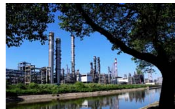
Sinopec Shanghai Petrochemical Company Limited
